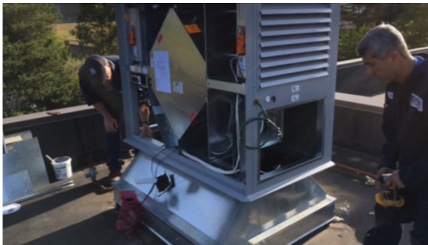
Installation of the Ventacity HRV
