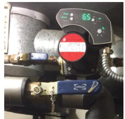
pump to match the needs of the system, adapting to pressure or flow requirements and reducing power when demand is lower. The energy-efficient electronically commutated motor (ECM) saves energy no matter how the circulator pump is operating.
