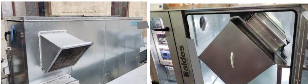
Figure 5: Photo of Mid Tier HRV products installed and showing internal components.
