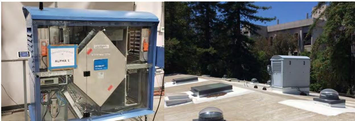
Figure 3: Photo of a VHE HRV product internal components and as installed.
