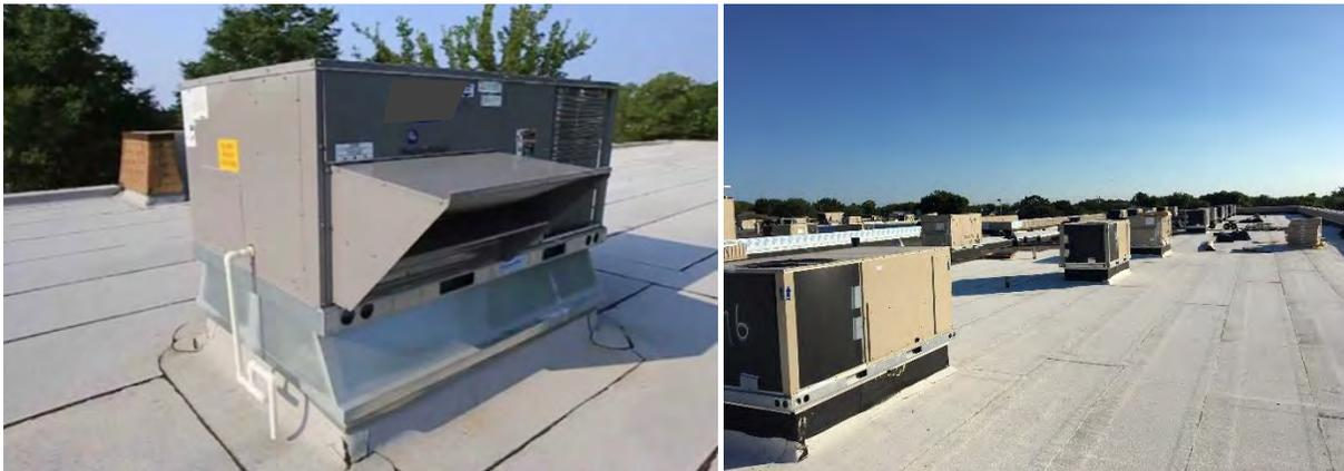
Figure 9: RTU packaged unit installations on rooftops.
