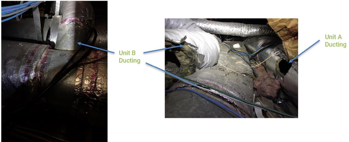
FIGURE 12: DUCTWORK PHOTOGRAPHS SHOWING LEAKING/DISCONNECTED DUCTWORK
