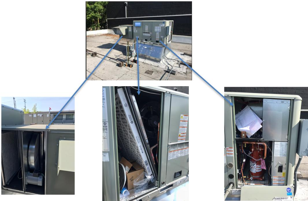
FIGURE 11: UNIT B CONFIGURATION INCLUDING BOLT-ON ERV
