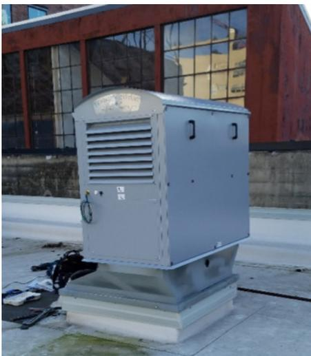
As shown in the photo to the left, the existing curb for the original RTU was relatively small. The curb adapter required careful redirection of the HRV airflow without imposing significant external static pressure. As in all exterior ducting, careful attention to detail in airflow restrictions, air-sealing, and insulation are required to enable optimal performance of the ventilation system.
