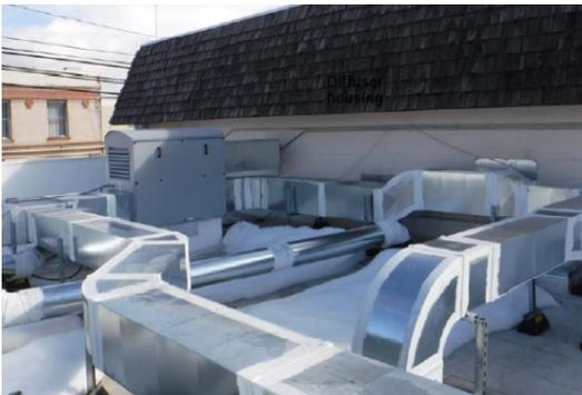
The conversion project added ventilation-zone control dampers to ensure that the ventilation air in the office space was not affected by the ventilation and exhaust movement in the storage/garage space. As exterior ducting heat loss significantly affects the performance of an HRV system, this system characteristic has an adverse impact on the energy performance of the ventilation system overall.
