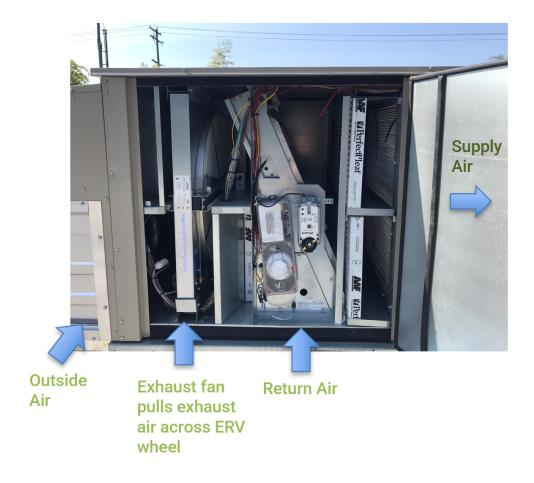
FIGURE 9: UNIT A ERV AND AIRFLOW PATH
