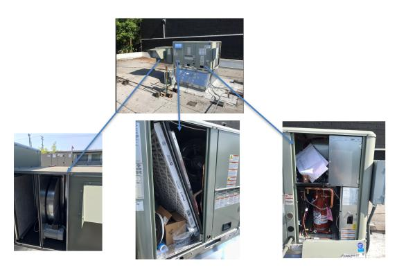
FIGURE 11: UNIT B CONFIGURATION INCLUDING BOLT-ON ERV
