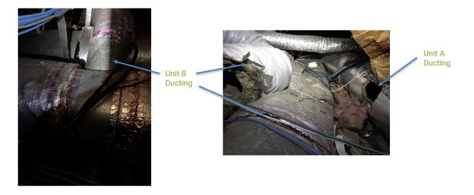
FIGURE 12: DUCTWORK PHOTOGRAPHS SHOWING LEAKING/DISCONNECTED DUCTWORK
