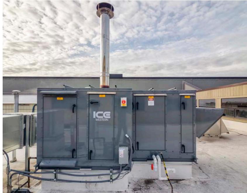
*Bend, OR* — Condensing RTU with evaporative air conditioning feedwater piping visible. Because of the high efficiency of this unit, moisture in the flue gases is condensed and this condensate needs to be managed and disposed of appropriately.
