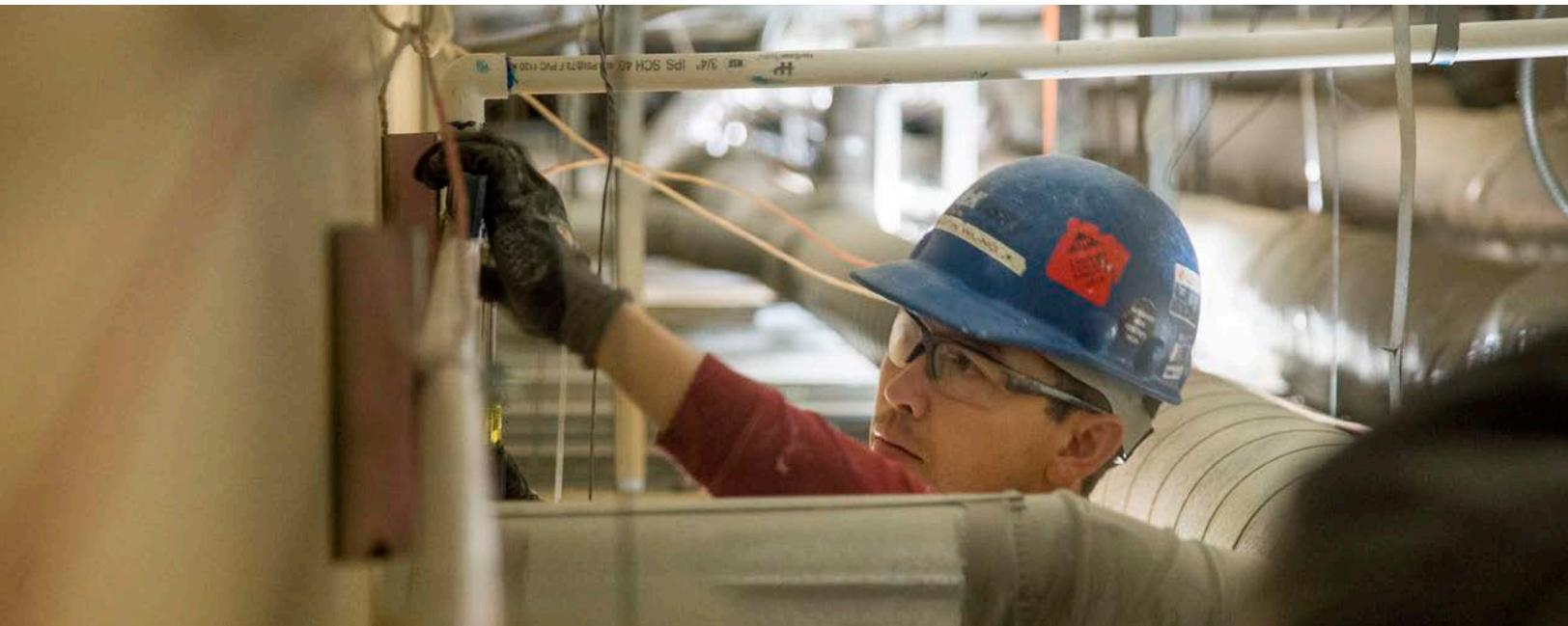
*Renton, WA* — PVC condensate line installation at a 2% (1/4-inch per foot) slope utilizing conventional hangars and unistrut supports.
